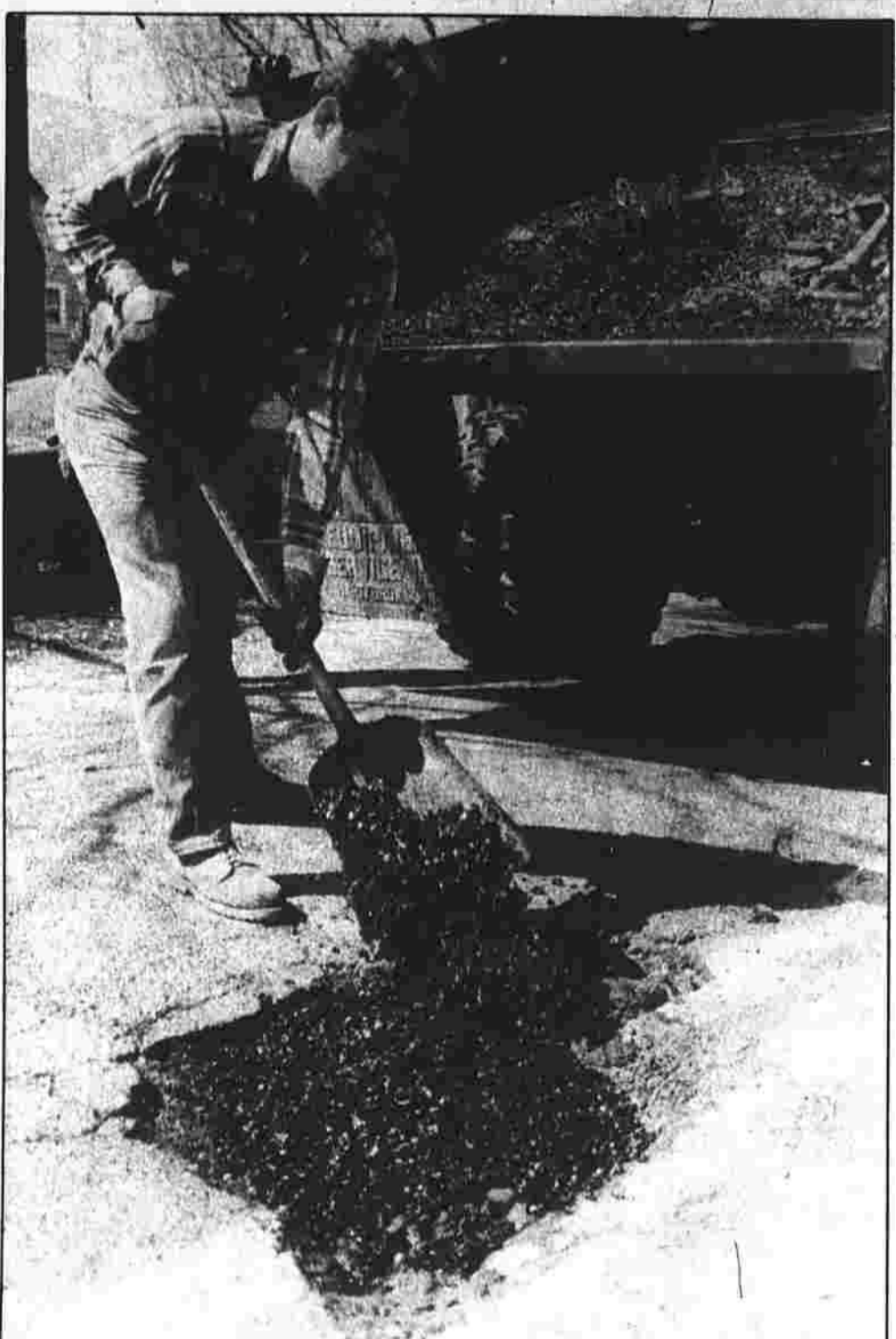
John Banas of Manchester, 29, a town Highway Division employee for 14 months, fills a pothole Wednesday afternoon on Irving Street.
